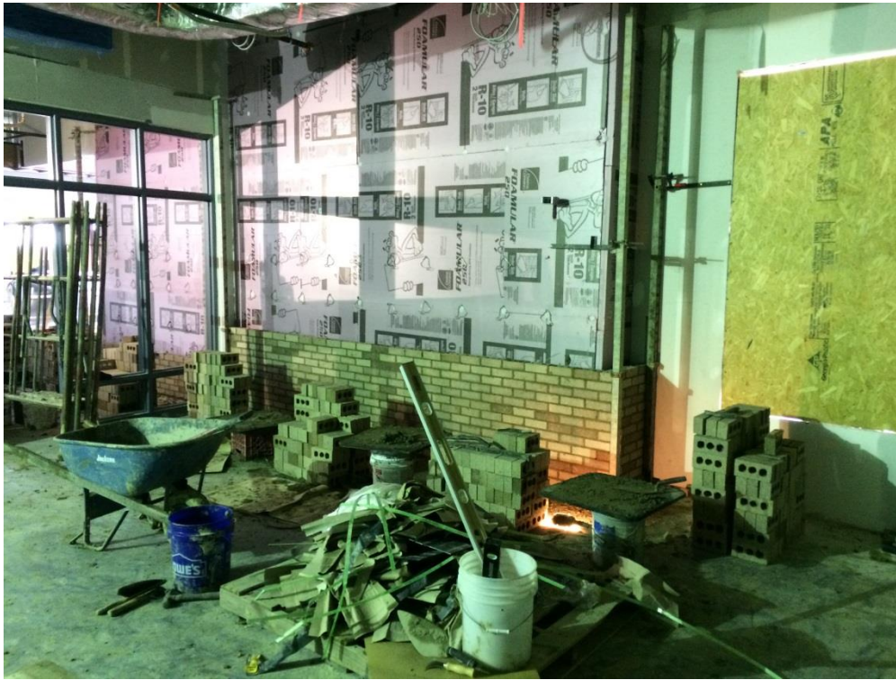
Project Site on February 6, 2019 View inside of the interior brick in the Community Room.
