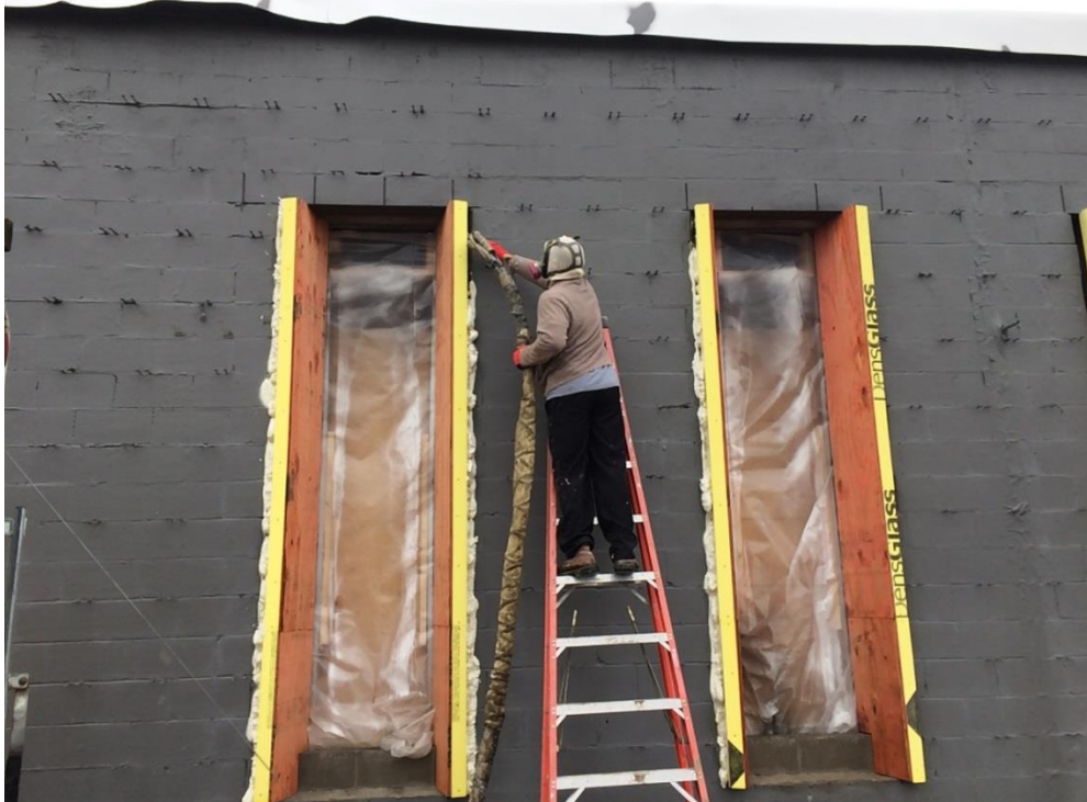
Project Site on February 6, 2019
