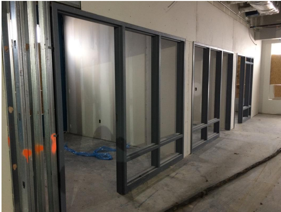
Project Site on February 6, 2019
