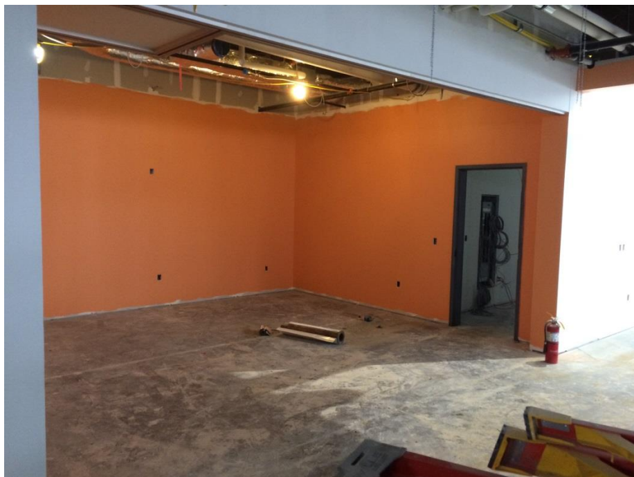
Project Site on February 6, 2019
