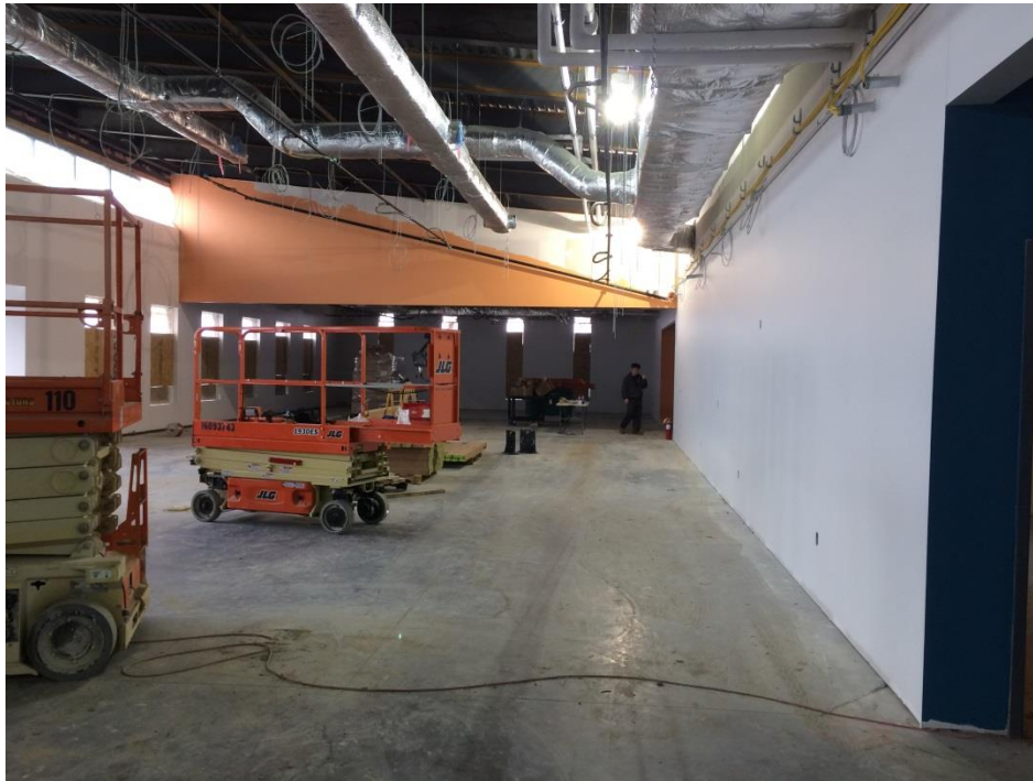
Project Site on February 6, 2019 View inside looking east showing the Children's Area.
